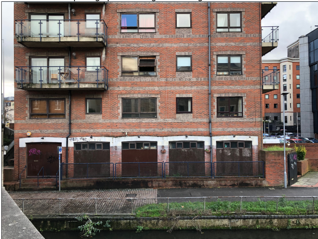
View of basement level façade from Kings Road Bridge
